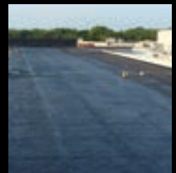
ASPHALT/BUR/ GRANULAR CAP SHEET
